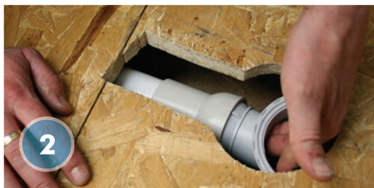
Boarding lowered between joists
